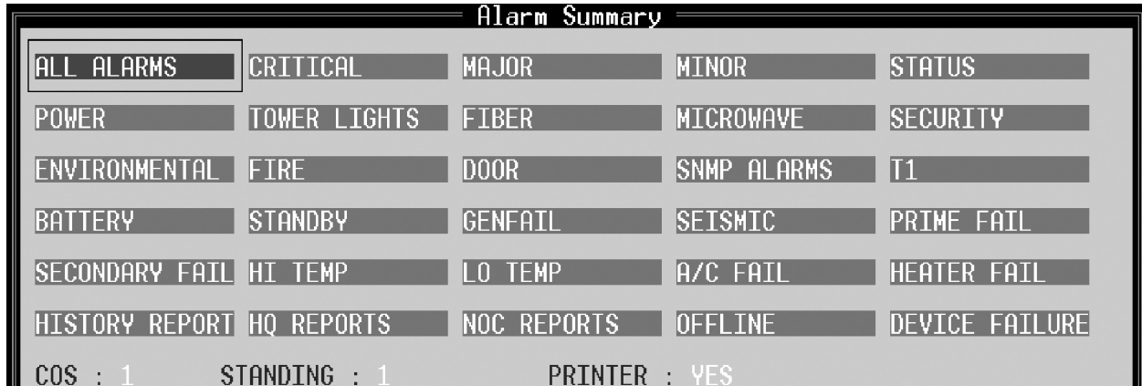
Fig. 16.4 - Upper portion of alarm summary screen shows 30 alarm windows.
