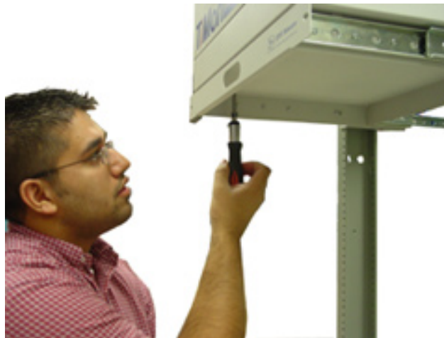
Fig. 1.5 - Secure the T/Mon NOC by inserting the two mounting screws from below
